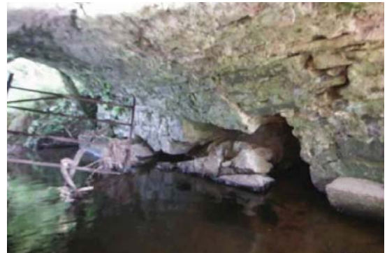
Figure 18. Abutment component rated condition '5' in a structure with an overall condition rating of '5'.
