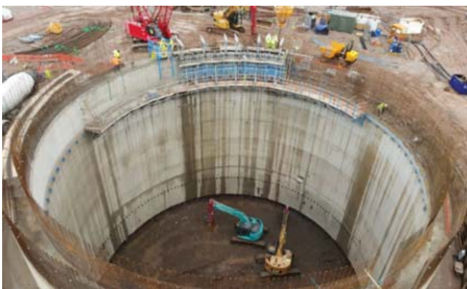
Figure 1 30 m diameter reinforced concrete caisson at Anchorsholme Park, Blackpool, constructed by Ward and Burke Construction
