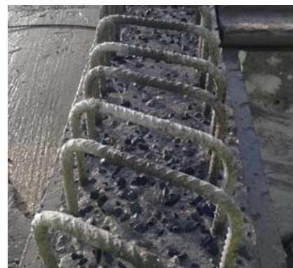
Figure 2. Interface Reinforcement close to beam ends showing a Rough Surface Finish (Source - Banagher Precast Concrete).
