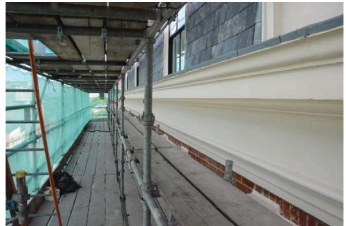
Figure 10. Finished Surface Following Installation of Cathodic Protection System. Note no Evidence of Anodes or Cabling which was Imperative for this Listed Structure.
