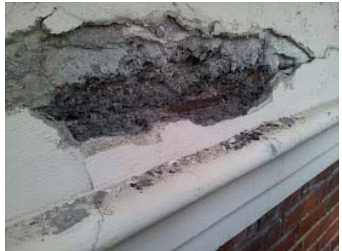
Figure 4. Subsequent Breakouts around the Horizontal Cracking Revealed the Presence of a Corroding Steel Member
