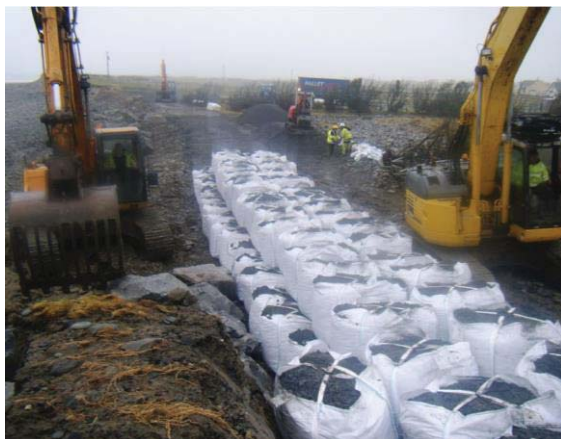
Figure 3 Emergency repair work being undertaken on the coastal embankment (photo provided by Clare County Council)
