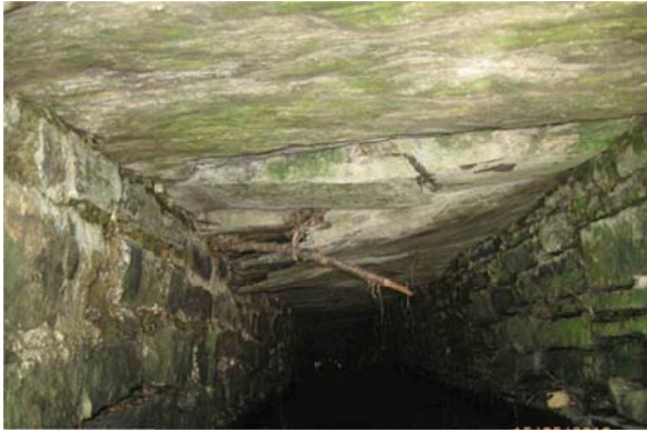
Figure 7. Typical 'clapper' bridge deck arrangement.
