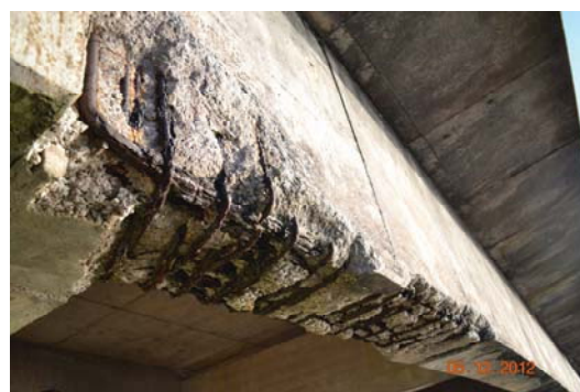
Figure 4. Typical concrete spall with exposed and corroded reinforcement.
