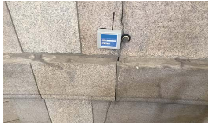
Figure 9. Installation of a MCM on a Masonry Crack
