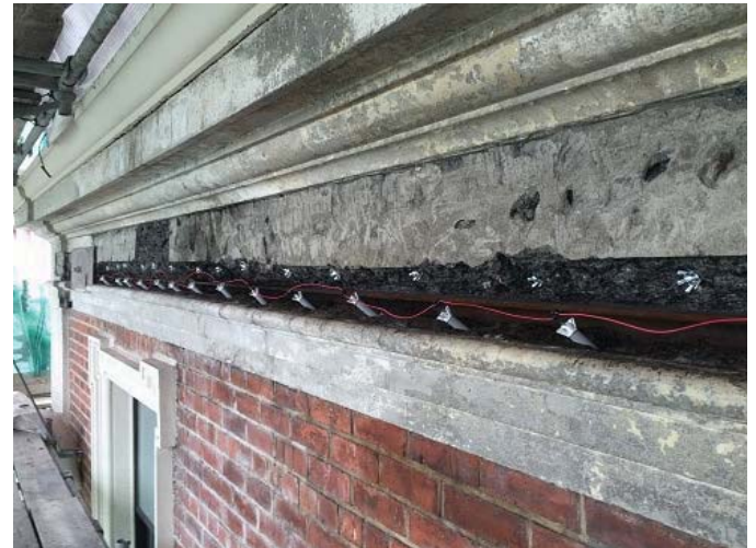
Figure 6. Hybrid Anodes in Preparation for Installation along the Kildare Street Elevation
