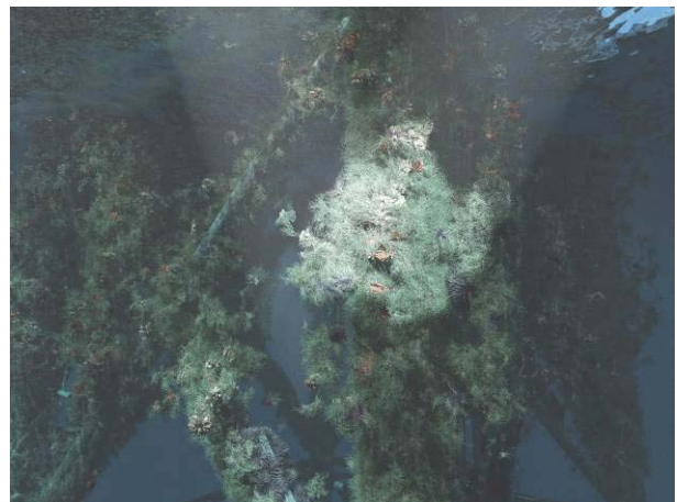
Figure 4. Rendered image of marine growth colonised structure taken by the left camera of the virtual stereo system.
