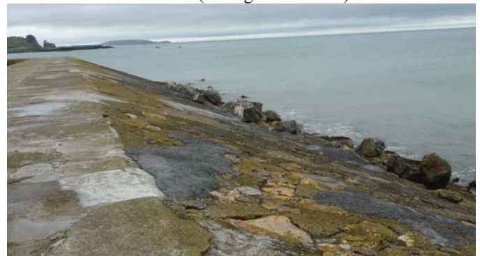
Figure 7. Repairs in the revetment at Howth Harbour's East Pier.
