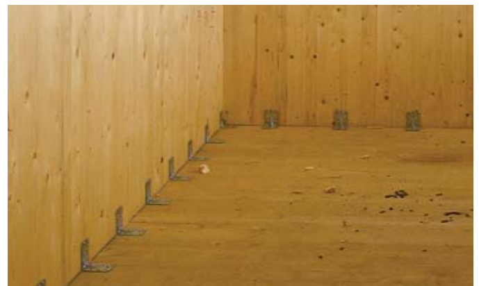
Figure 8. CLT wall floor connection – Murray Grove [13].
