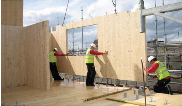
Figure 3. Platform construction – Murray Grove [13].
