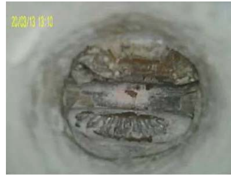
Figure 6. Image from the PTSI showing Tendon T47 fully grouted and corrosion free.
