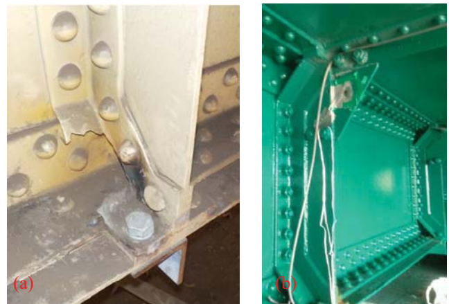
Figure 6. Stiffeners on rail-bearers section loss (a) and strain gauge placement (b)
