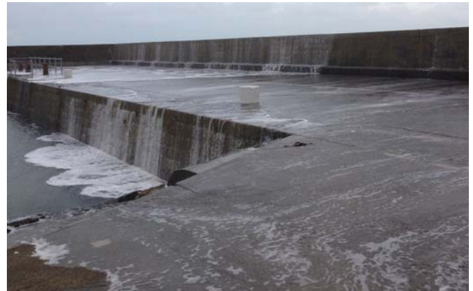
Figure 4. Overtopping during an extreme event at Howth Harbour's East Pier.
