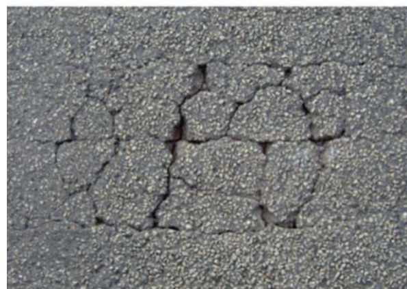
Figure 2 Damage to asphalt surfacing
