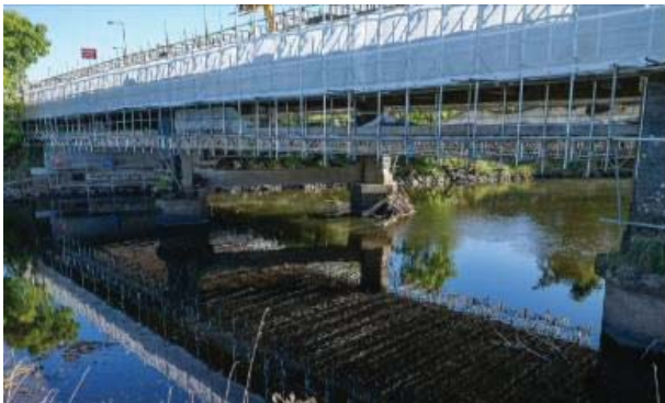
Figure 8. Installed Scaffold.
