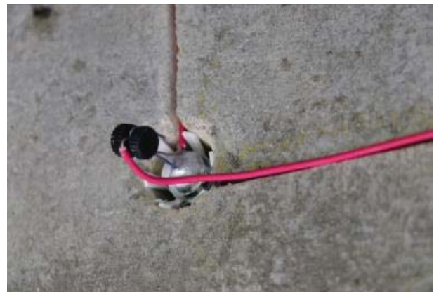
Figure 7. Partially Installed Anode.
