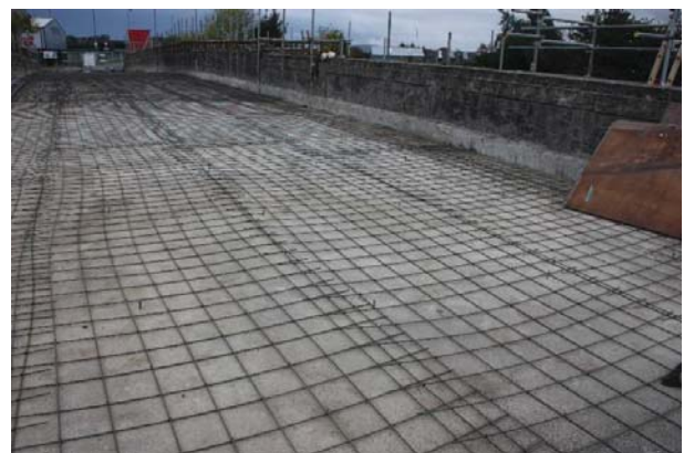
Figure 4. placement of the BFRP mesh prior to the pouring of the lightweight aggregate concrete
