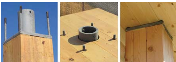
Figure 18. Floor column connector [29].
