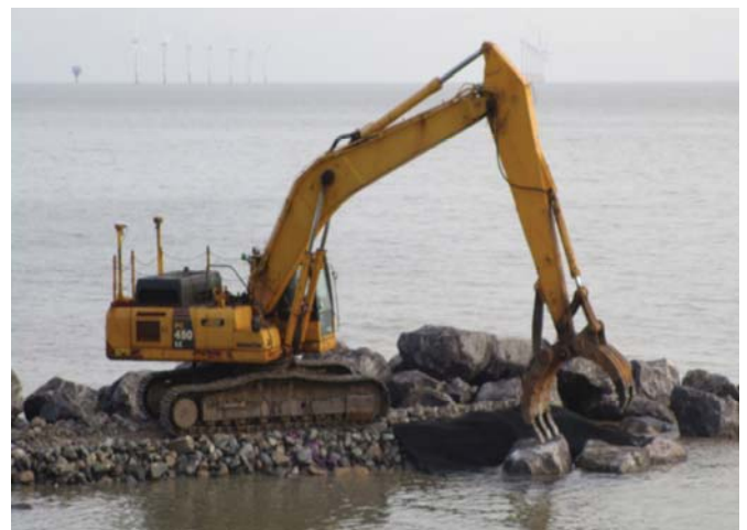
Figure 5 Excavator surveying section of rock groyne”
