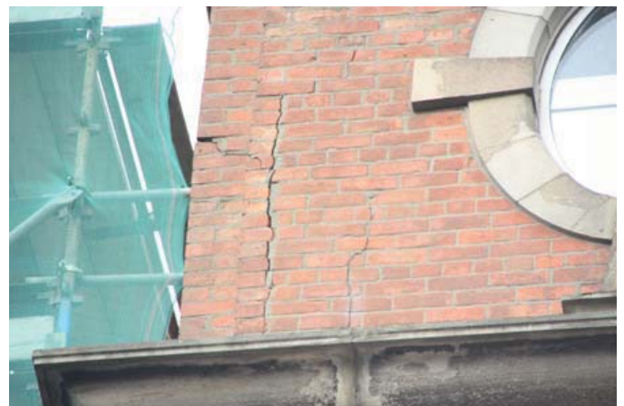
Figure 1. Cracking on Masonry Façade Attributed to Steel Corrosion. Often Wrongly Identified as Structural Movement of Foundations etc
