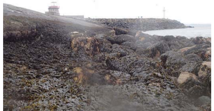
Figure 8. Undermining at the toe of the structure.
