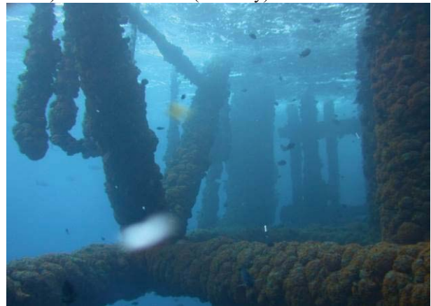
Figure 3. Real world structure affected by marine growth.
