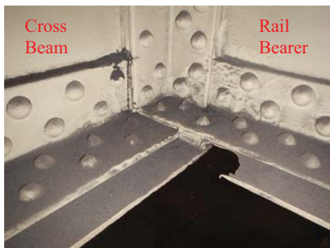
Figure 3. Section loss for critical rail bearer
