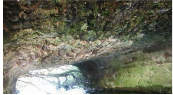
Figure 17. Deck (arch barrel) component rated condition '5' in a structure with an overall condition rating of '5'.
