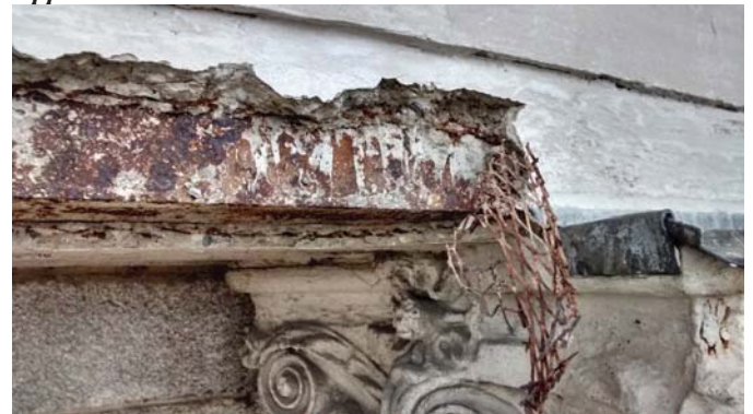
Figure 3. Corrosion of the Steel Tension Band at the Base of the Dome and Associated Concrete Spalling
