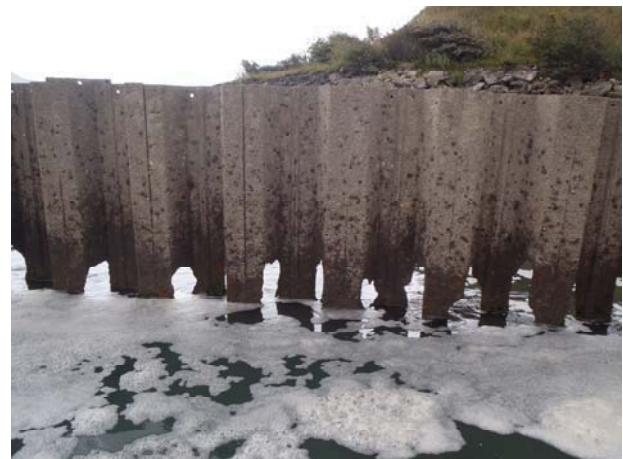
Figure 8. Holes in existing eastern sheet-pile wall subjected to direct flow from weir
