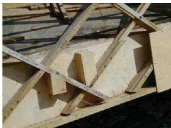
Figure 7: Gridshell laths bolted to plywood perimeter
