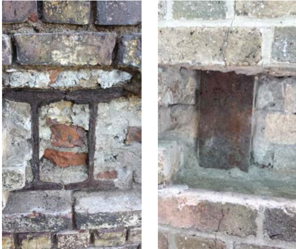
Figure 2. Corroding Steel Frame Filled with Porous ‘Builders Rubble’ on an Irish Heritage Structure. Note Vertical Cracking on Brickwork Façade over Steelwork
