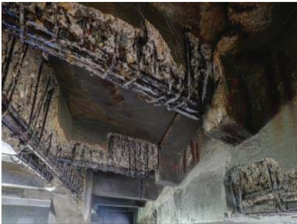
Figure 5. Concrete Elements Prior to Repair.
