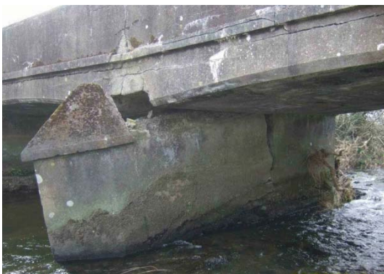
Figure 16. Intermediate pier component rated condition '5' in a structure with an overall condition rating of '5'.
