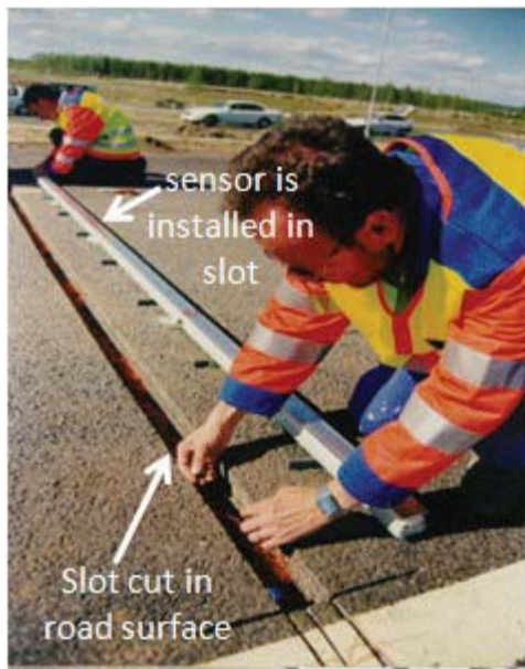
Figure 1. Installation of WIM Sensor.
