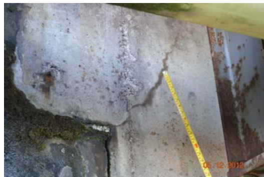
Figure 3. Typical inclined crack from the re-entrant corner at half-joints.
