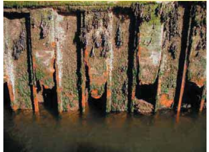
Figure 6. Accelerated Low Water Corrosion, ALWC - International Navigation Association [6]
