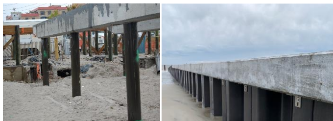
Figure 7. Pipe pile and sheet pile installations (Creative Composites Group and CMI/Strongwell).
