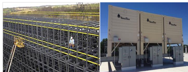
Figure 2. Stick-built (under construction) and Frame-type Cooling Towers. (Strongwell, Creative Composites Group/Tower Tech)
