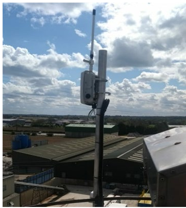
Figure 7 LoRa gateway installed at 50m altitude.
