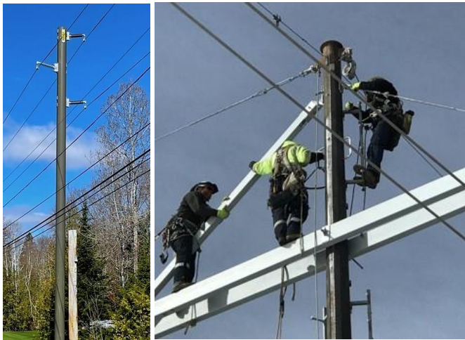
Figure 6. Round pultruded pole and pultruded cross-arm attachment (Creative Composites Group and PUP Inc).
