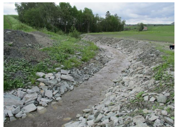
Figure 10. Erosion protection near to Esp quick clay landslide near Trondheim [2]
