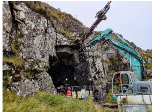
Figure 9: The 24T drilling rig at northern portal.
