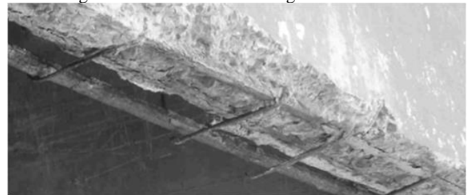
Figure 3 - Exposed shear reinforcement along the bottom of RC bridge beams [3]
