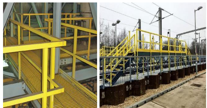
Figure 5. Pultruded Stairways and Platforms (Strongwell and Creative Composites Group)
