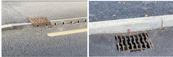
Fig 5(a) Linear kerb drain; (b) Kerb and gully
