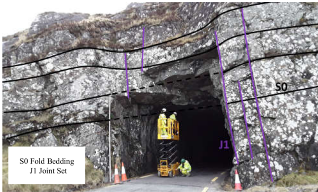
Figure 5: View of the northern portal. Note the size of the potential blocks hanging from the roof entrance and west wall.
