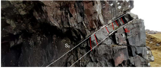
Figure 4: View of the northern portal west wall. Fold bedding (S0) intersecting the near-vertical cleavage (S1)
