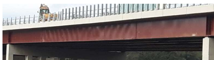
Figure 1. Observed deformations in the web plate of the N80-S1 River Slaney bridge girders
