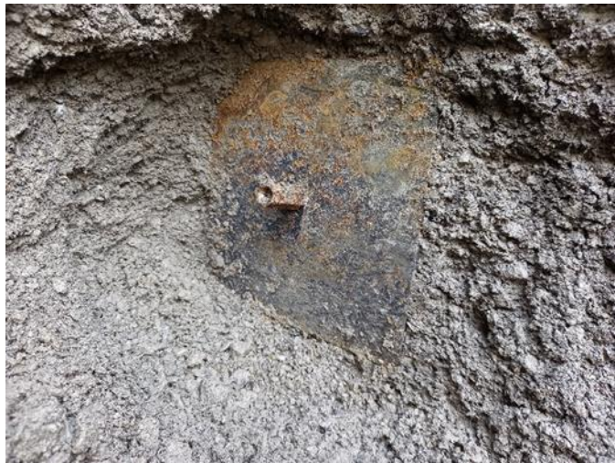
Figure 17. Exhumed Anchor 28.
