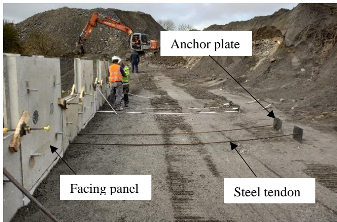
Figure 8. Construction of wall, including installation of anchors.
