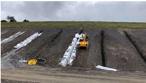
Figure 1: Counterfort drains
