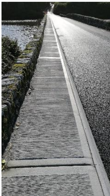
Figure 4. Typical concrete footpath to avoid cracking caused by pavements drying out over time.
